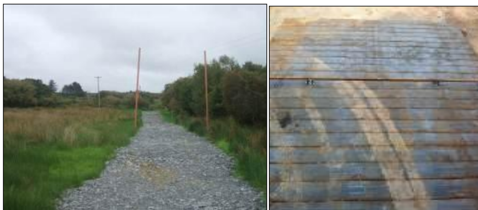
Figure 7.5: Temporary Stone Road and Wooden Sleepers
