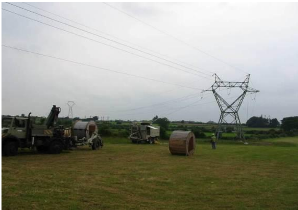
Figure 7.15: Typical Stringing Equipment
