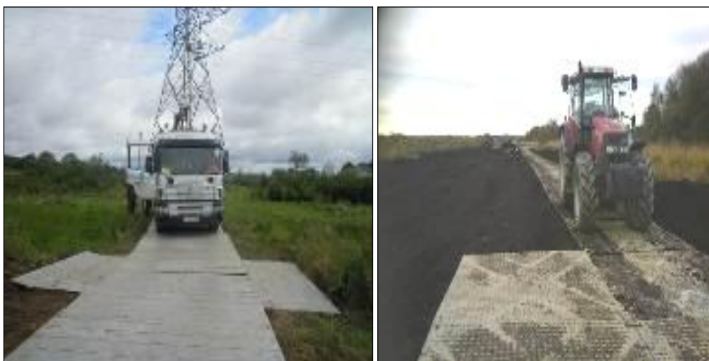
Figure 7.4: Temporary Aluminium and Rubber Panel Tracks
