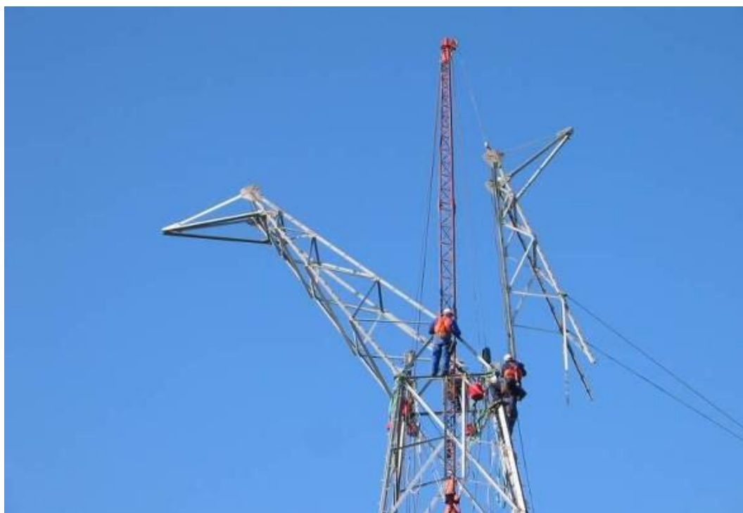
Figure 7.9: Lower Part of the Tower Head being dropped into Position
