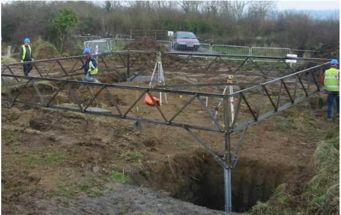
Figure 7.7: Photograph of Setting Template being prepared for Final Concreting
