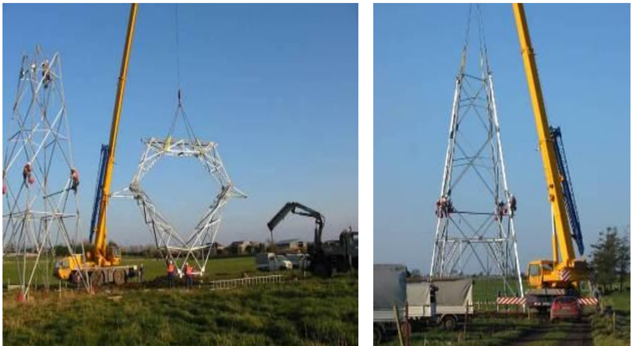
Figure 7.10: Tower Erection by Mobile Crane
