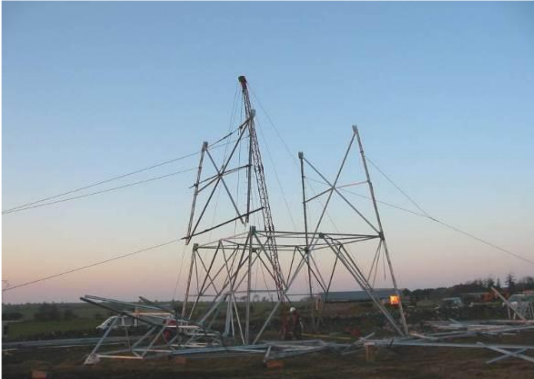
Figure 7.8: Derrick Pole at Tower Base
